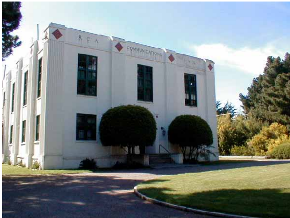
The KPH building as it sits today. We will take a tour of this building.
