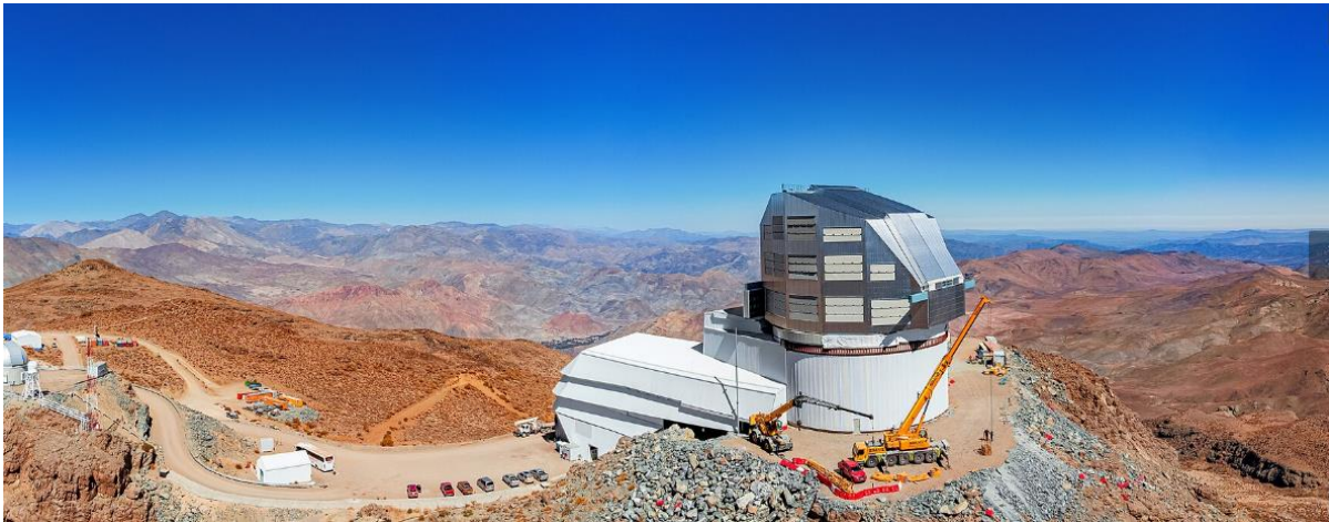
Construction progress as of 2022
